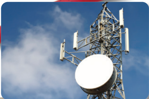
WIRELESS CELL TOWERS
